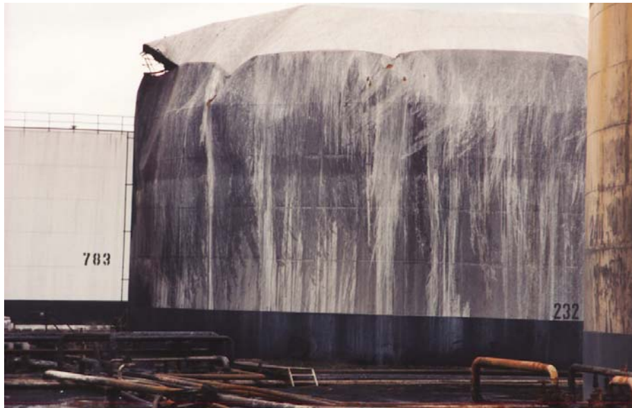
Fig. 2: Separation of roof-wall junction of a cylindrical tank with fixed roof
