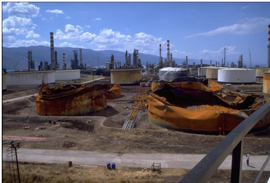
Fig. 3: Post-earthquake fire damage of the naphtha tanks at the Tupras Refinery
