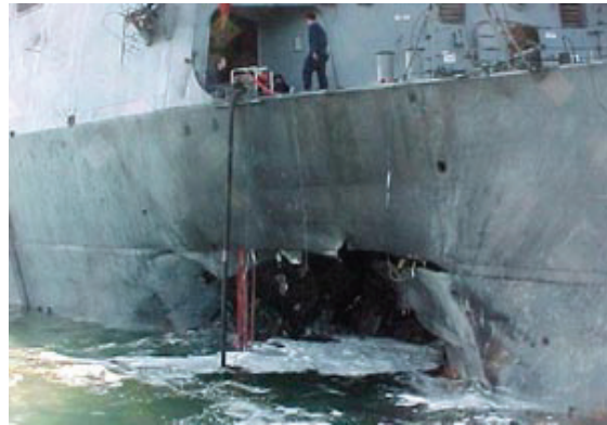
Figure 2 USS Cole nearby external explosion on water surface
