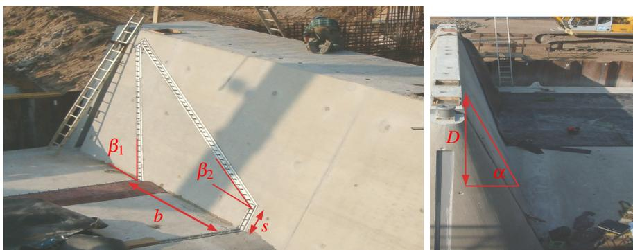
Figure 8: Side dam with a sketch of the rubber fixation
