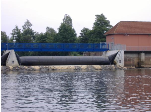
*Figure 1: Water filled inflatable dam near Marklendorf*
