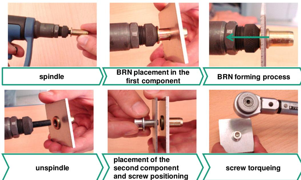
Fig.3: Installation process of a traditional blind rivet nut (cf. [3])
