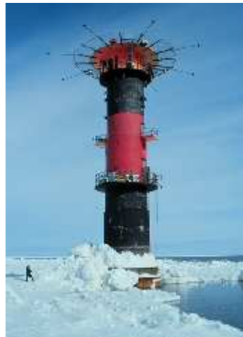
Figure The lighthouse Norströmsgrund is located in the Gulf of Bothnia, about 65 km southeast of Luleå in Sweden [3]. It shows the accumulated ice after crushing.
